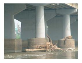
Figure 4 Debris trapped in front of the bridge piers
