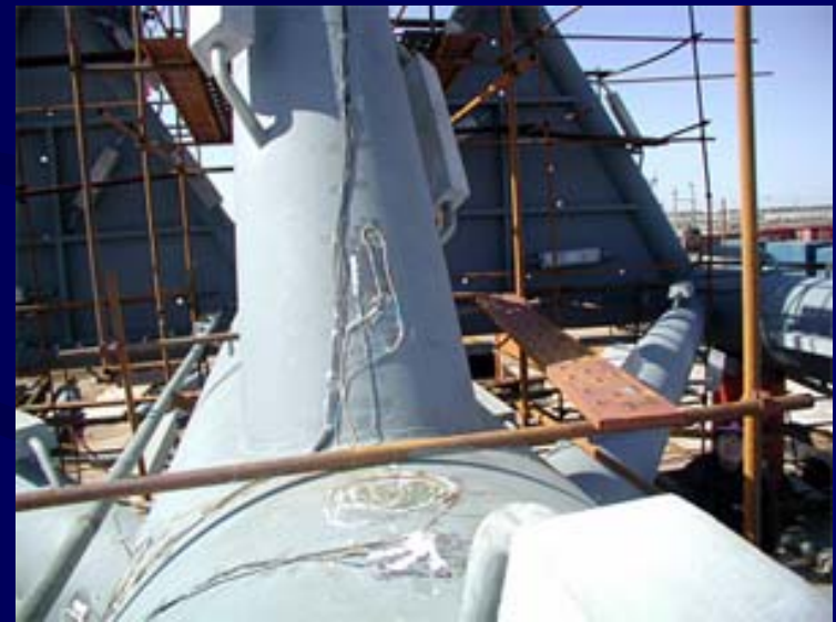
Fig. 22. Sensors installation in oil production platform
